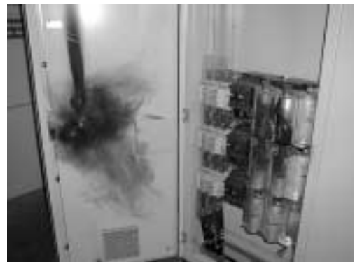
Figure 5 - What uncontrolled resonance may do
