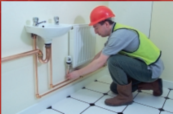
An example of a copper system installed by using push-fit fittings for connections made in seconds.
