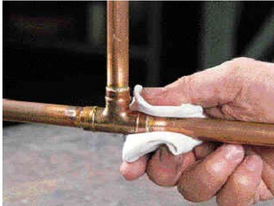
Figure 12 – Removal of excess flux
