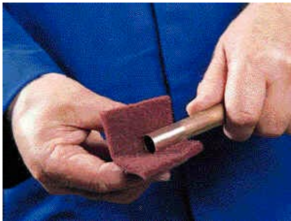
Figure 6 – Cleaning the tube end
