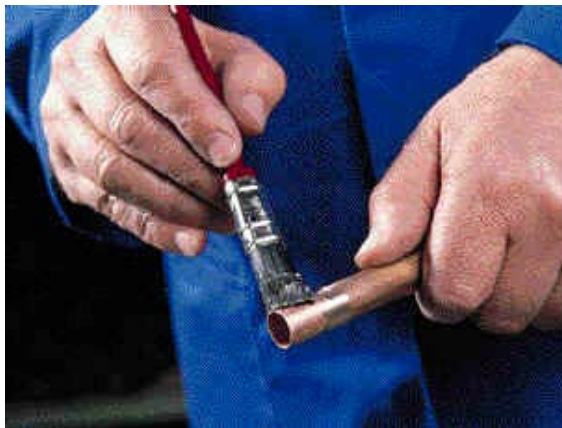
Figure 8 – Applying flux to the tube end
