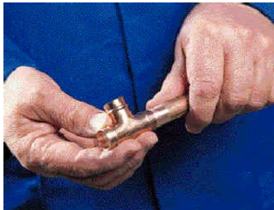
Figure 9 – Assembling the joint
