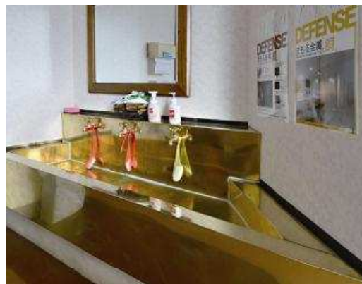
Antimicrobial Copper hand-washing station
