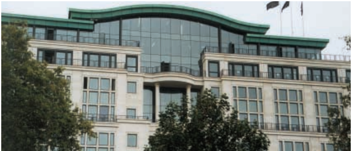
Globe House offices, London. Architect: GMW. Roofing Contractor: Richardson Roofing.
