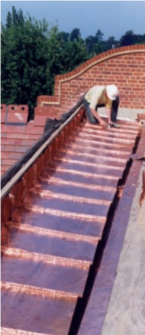
Copper roof installation at Linacre College, Oxford.
