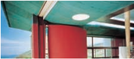
Baggy House, Devon. Architect: Anthony Hudson Architects. Roofing Contractor: Richardson Roofing.
