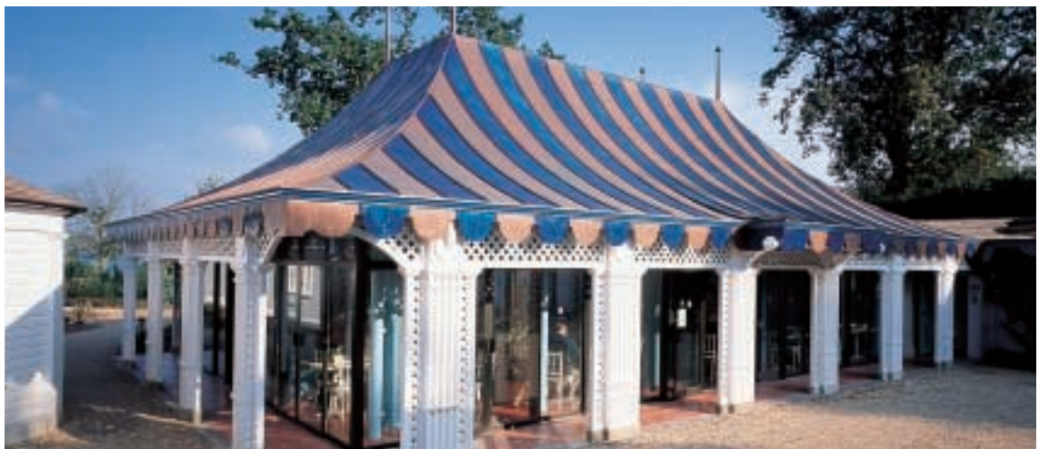
Nymans Garden, West Sussex. Architect: Winchester Design (Architects). Roofing Contractor: Wessex Roofing.
