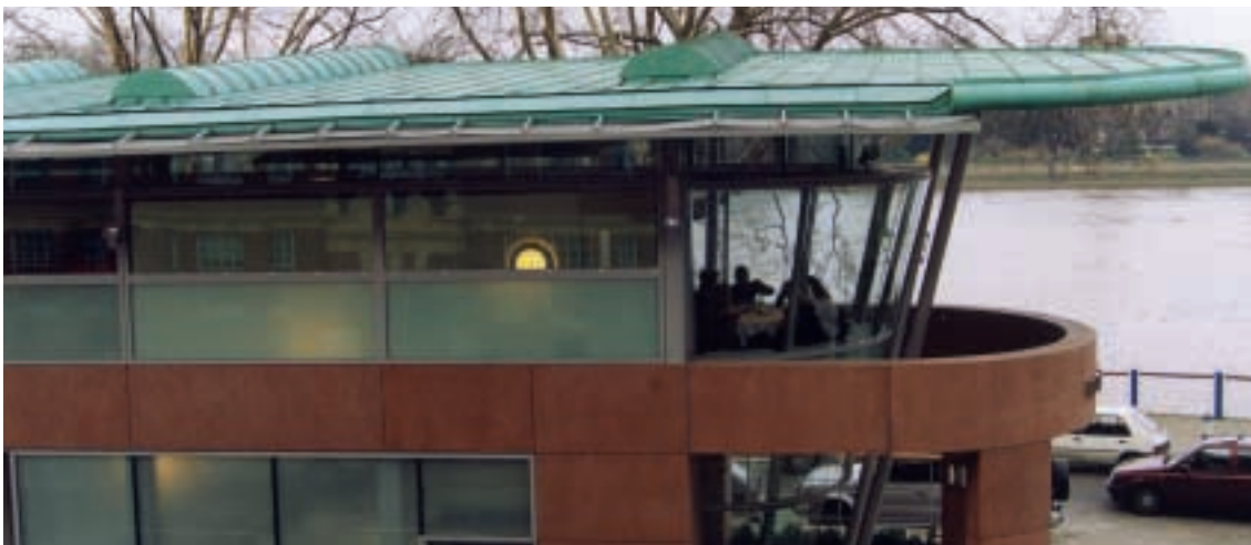
Putney Bridge, London. Architect: Paskin Kyriakides Sands. Roofing Contractor: Cotswold Metal Roofing.
