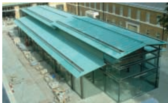
Duke of York's Headquarters, London. Architect: London Bloc Architects. Copper Contractor: T+P Lead Roofing.
