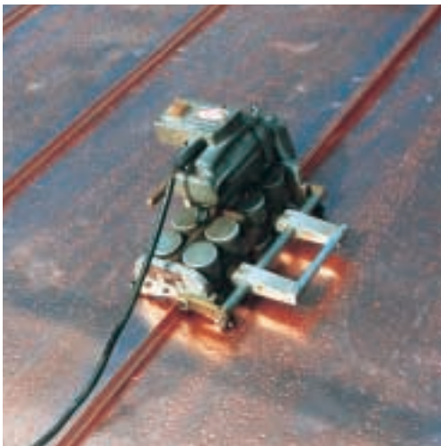
Mechanised seaming, Long Strip system.
