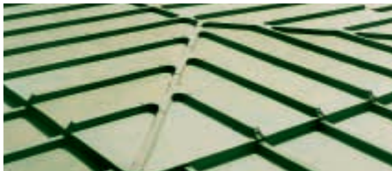
Traditional batten roll method.
