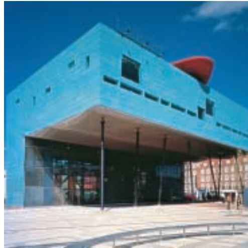
Peckham Library. Architect: Alsop and Stormer Architects. Copper Contractor: Cleveco.
