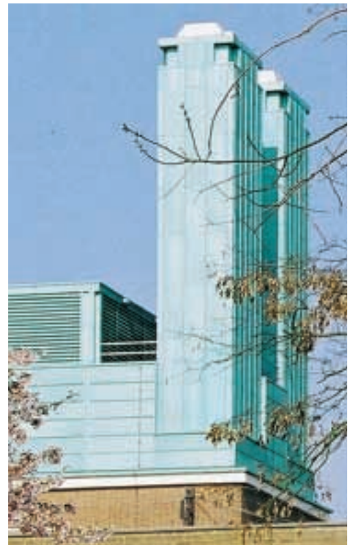
Department of Chemistry, University of Cambridge. Architect: Nicholas Ray Associates. Copper Contractors: Richardson Roofing & T R Freeman.
