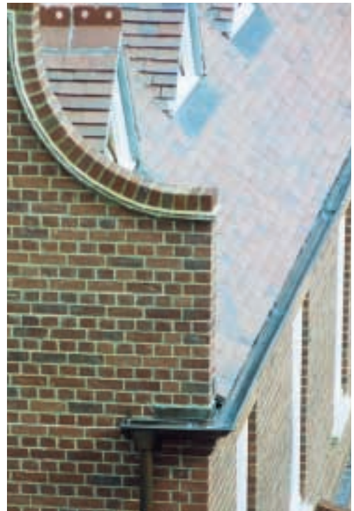
Copper gutters, downpipes, flashings and weatherings at Linacre College, Oxford (BREEAM Gold Medal). Architect: ECD Partnership. Roofing Contractor: Cotswold Metal Roofing.
