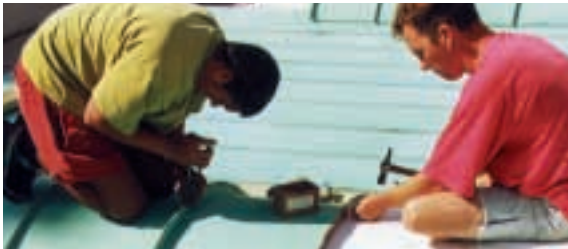
Installation of pre-formed curved trays.
