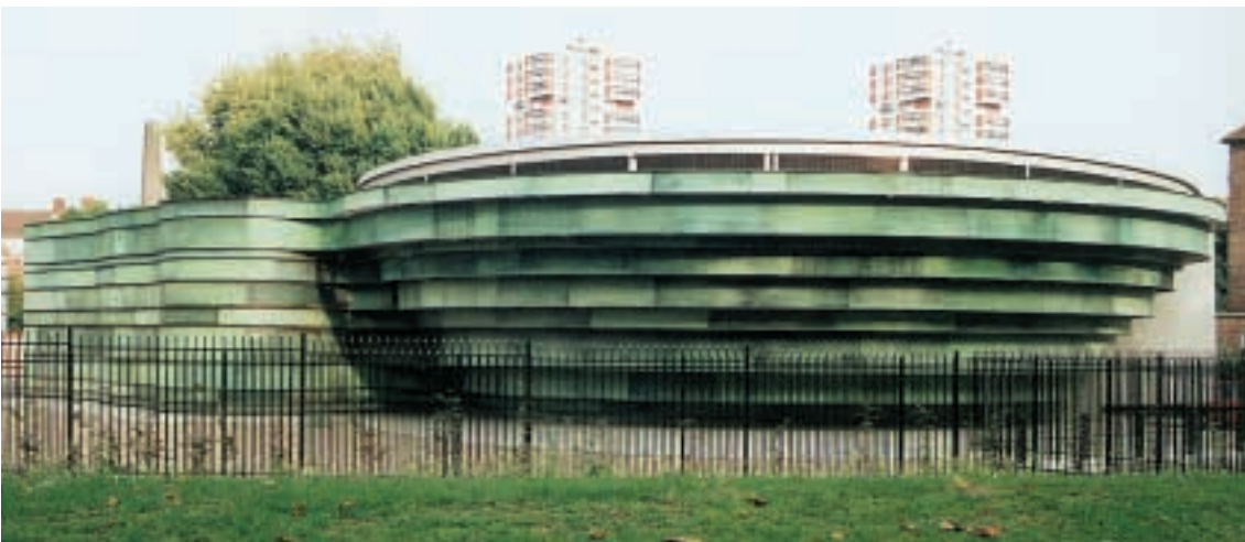
JLE Vent Shafts, London. Architect: Ian Ritchie Architects. Copper Contractor: Entech.
