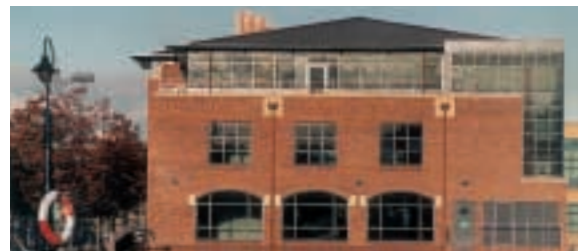
Profiled sheet roofing on commercial offices, Belfast.
