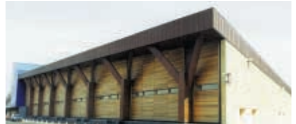
CRS Retail Store, Cardiff. Architect: GHM Rock Townsend. Roofing Contractor: Kelsey Roofing.
