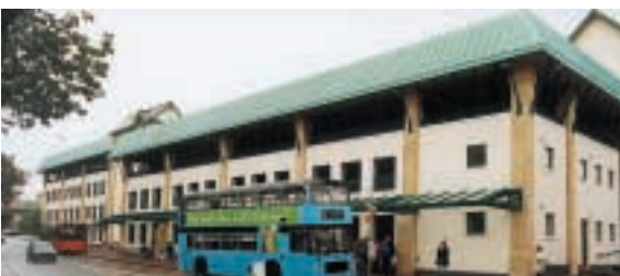
Multi-storey car park, Caernarfon. Designers: Adams Consulting Engineers. Roofing Contractor: Varla (UK).
