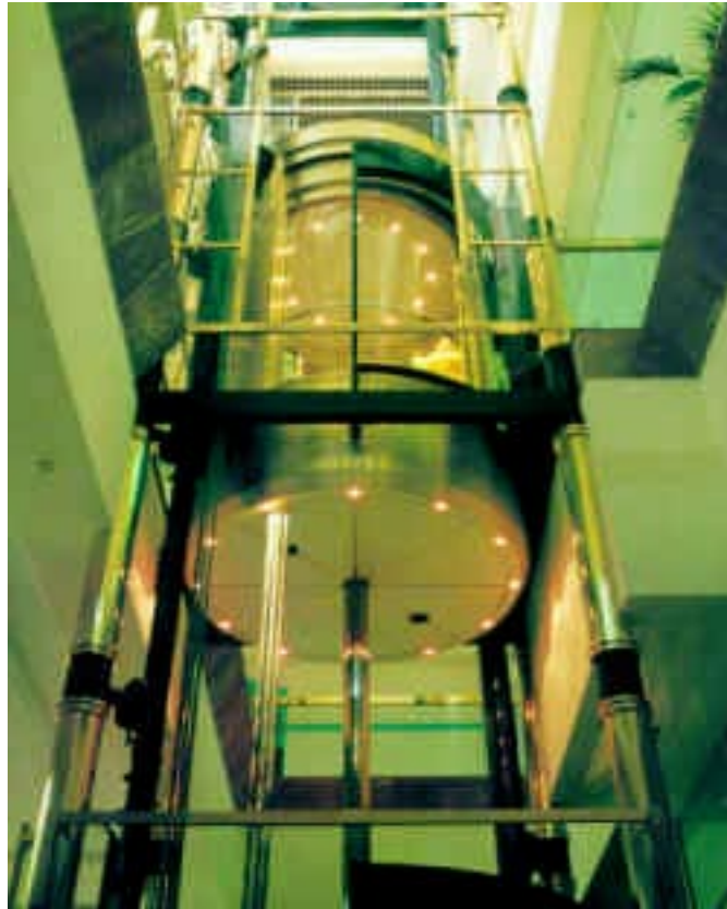
Decorative brass cladding to columns, safety screen and lift facade at Merry Hill centre, Dudley.
