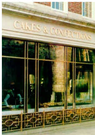
Window frames and infill panels at Betty's tea rooms York (Rileys (Metal Workers) Ltd)
