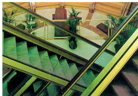
Arena handrails at Merry Hill Centre, Dudley (President Manufacturing Limited)
