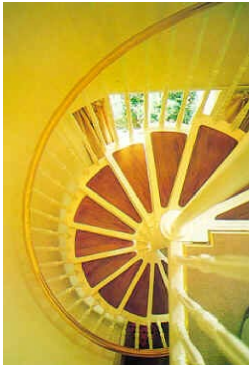
Brass handrails on a spiral staircase in a residential accommodation (County Forge Limited)
